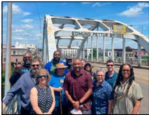
Crossing the Edmund Pettus bridge to feel the power of the great marches of the Civil Right
